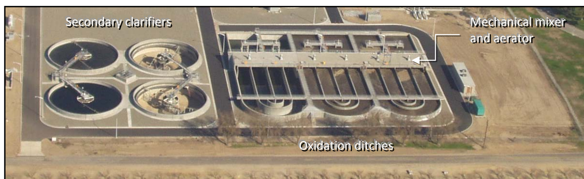
Figure 5.4: Example oxidation ditches and secondary clarifiers at a 10-MGD plant.
